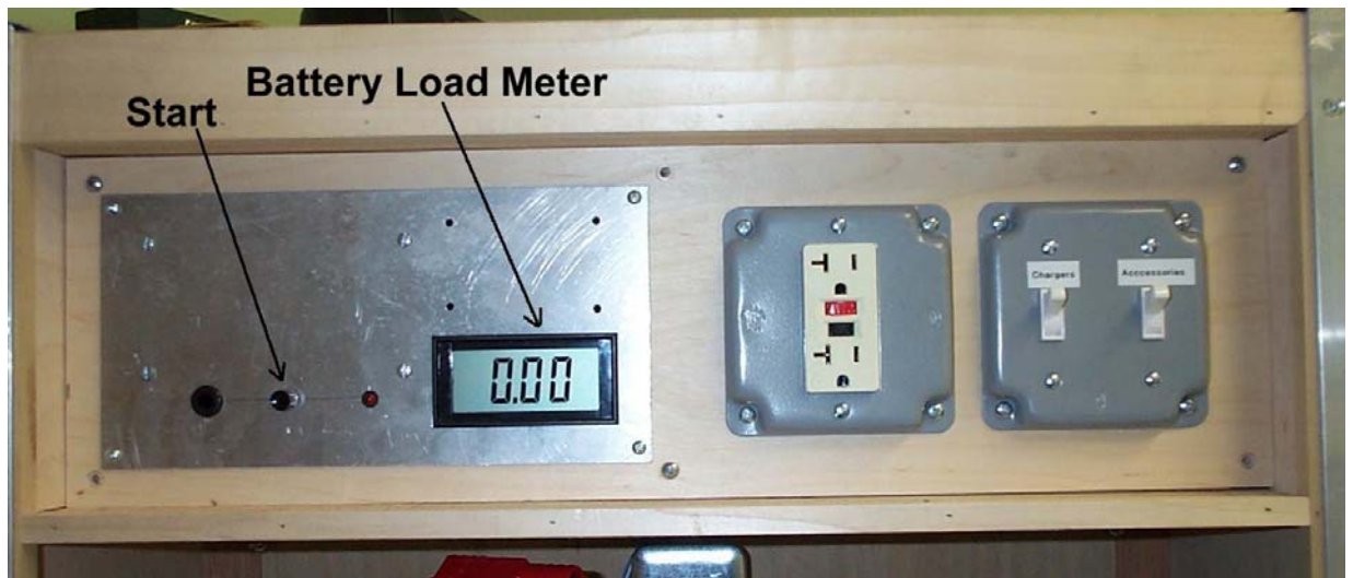
Photo S: Load Test Panel
